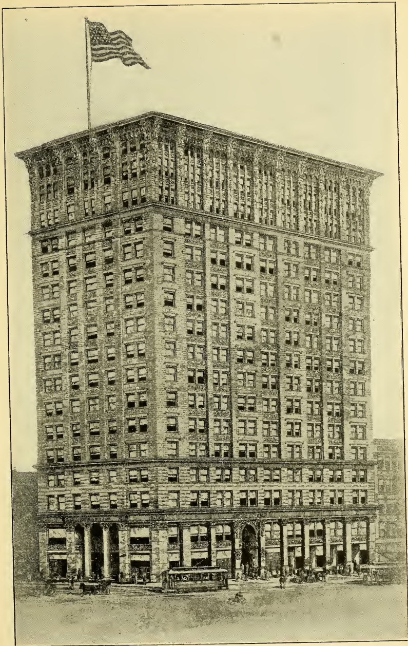
CANDLER BUILDING Junction Peachtree and North Pryor Streets
